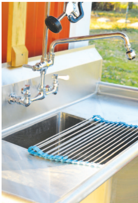
The author's adjustable-height washing sink, with detail showing the stainless steel grate that can be added to use it as a spray table.
